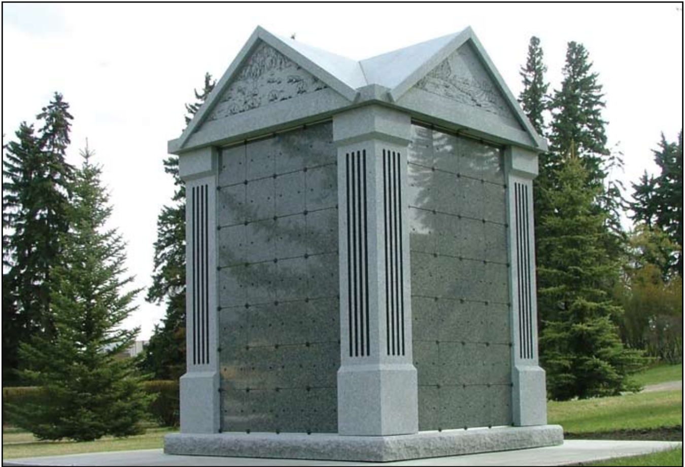
The S112 model installed at Union Cemetery for the City of Calgary.
